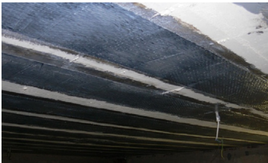
Fig. 3. Strengthening of reinforced concrete beams in Russia
