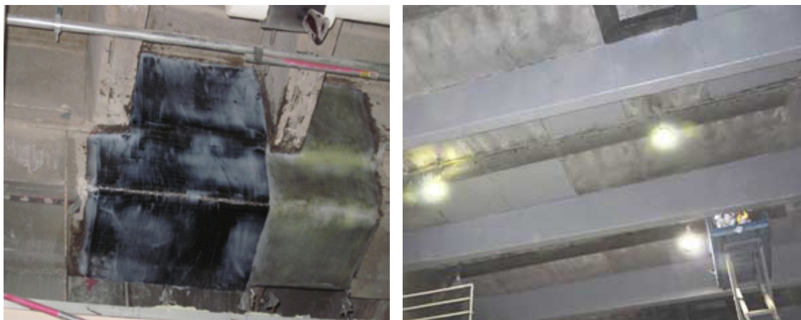
Fig. 2. An application of carbon fiber reinforced polymers in USA
