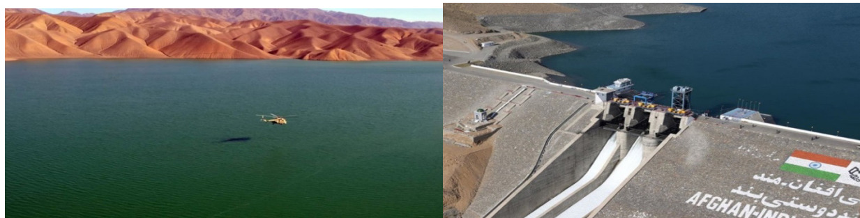
Fig.4. Salma Dam and reservoir [8, 9]
